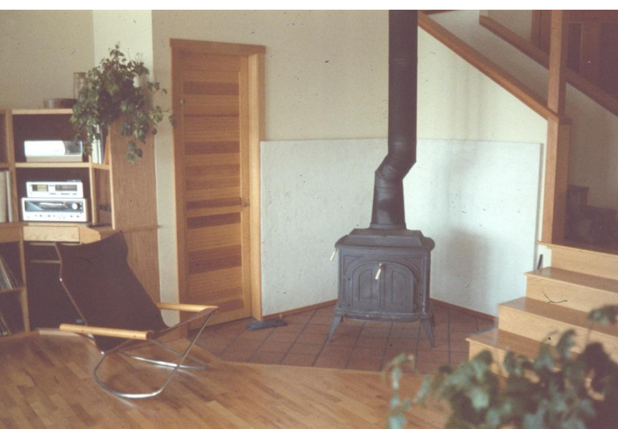
Wood stove as back-up heater (above)
