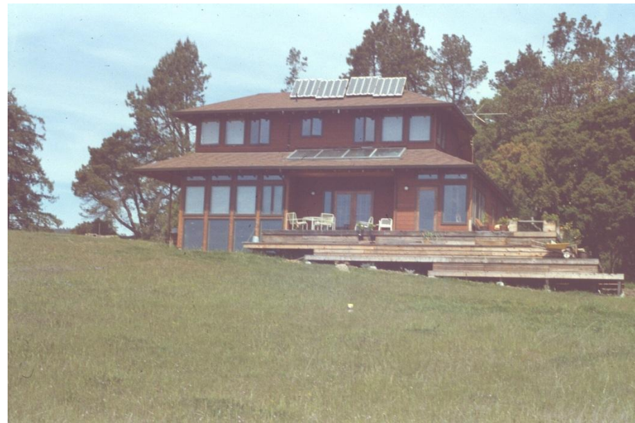
South view with solar PV on upper roof and integrated passive solar hot water heater on lower roof
